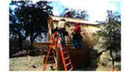
Building steel frame September 13, 2014
