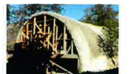
Curing the shell October 1-15, 2014
