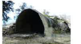
The completed shell October 17, 2014
