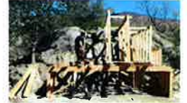
Building support frame August 31, 2014
