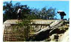
Building steel frame September 20, 2014
