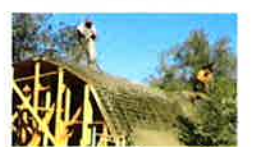
Cementing the shell October 1, 2014
