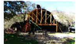
Completing support frame September 6, 2014
