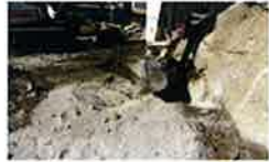
Digging the footings August 12, 2014
