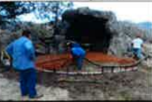
Pouring the floor December 4, 2014
