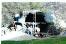
Creating artificial façade November 20, 2014
