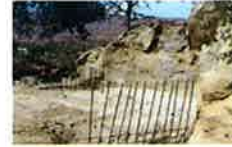
Tying the steel August 12, 2014
