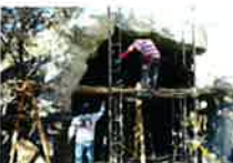
Spray painting base coat November 25, 2014
